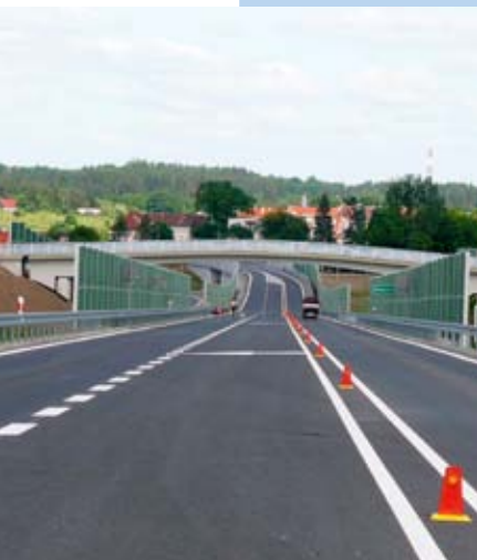
Construction of the bypass in Mrągowo
